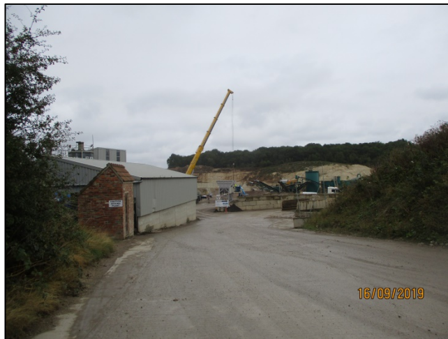
Internal haul road
